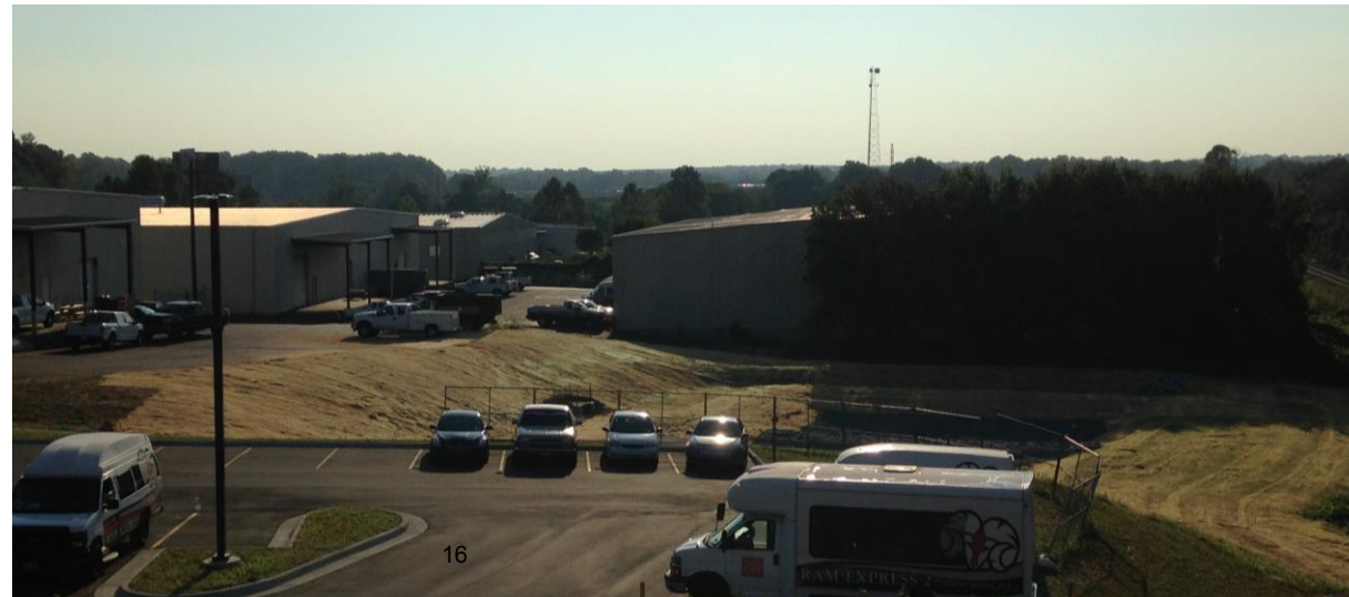
Storm Water Retention Basin and East Parking Lot
