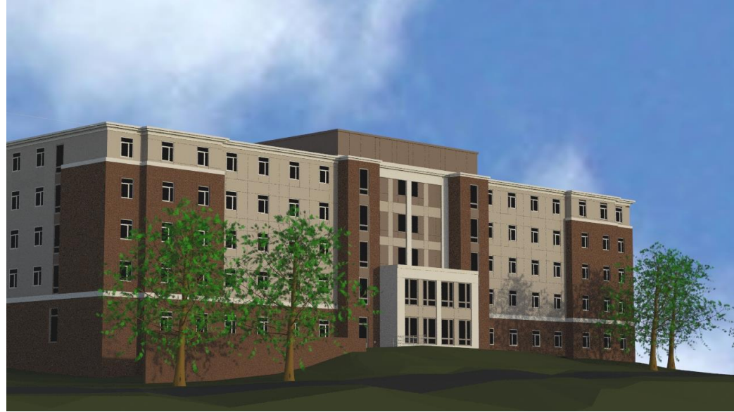
Rear View from Cromartie St.
