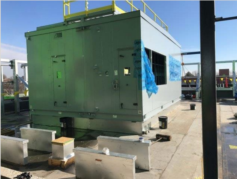
Heat Recovery Unit installation on Roof
