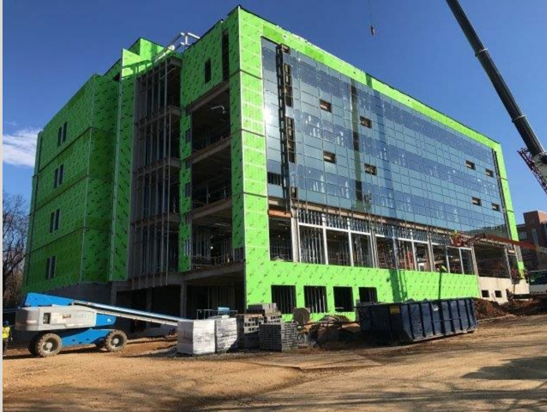
Curtainwall Glass installation
