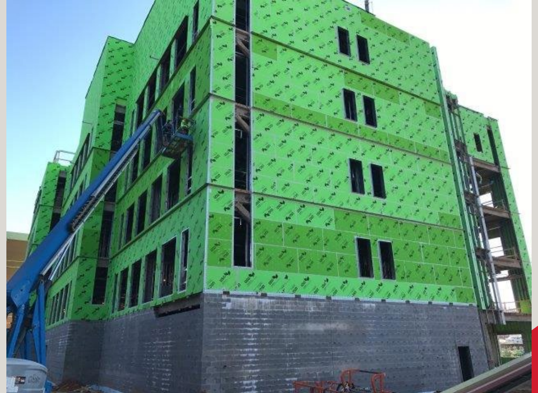
Exterior insulating sheathing installation
